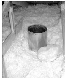
A core sample or cookie-cutter test involves taking at least three insulation samples and weighing them.
